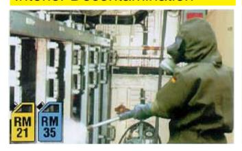
Detoxification and disinfection of buildings, shelters, etc. is carried out with help from dry steam of 210°C. A non aggressive decontamination agent, i.e. RM 21 or RM 35, can be added.
